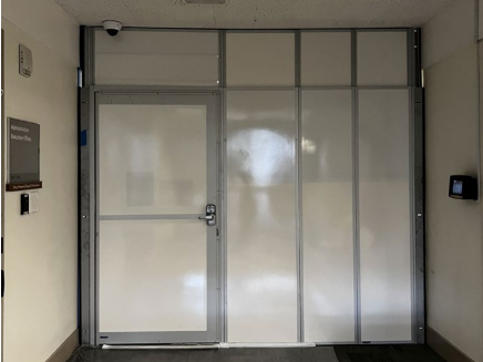
Temp Wall for SPC4D Corridor Work
